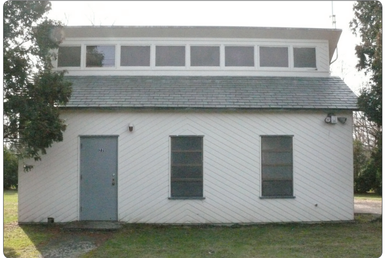
The unmanned and remote Stanley Street lift station is under constant surveillance thanks to AlarmAgent.com
